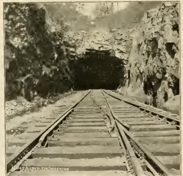
EASTERN ENTRANCE TO THE OXFORD TUNNEL ON THE D., L. & W., SHOWING TRACKS CONVERGING.
